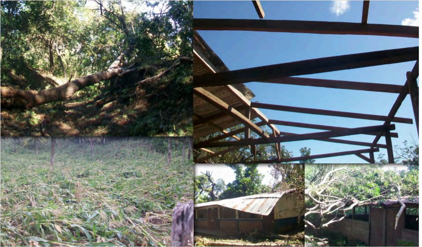
Extreme weather events are not new to Nicaragua, but two Cat 4 hurricanes in the matter of two weeks? These photos were sent to us from our partners at the El Porvenir Coffee Co-op in which plants and infrastructure were both badly damaged.
